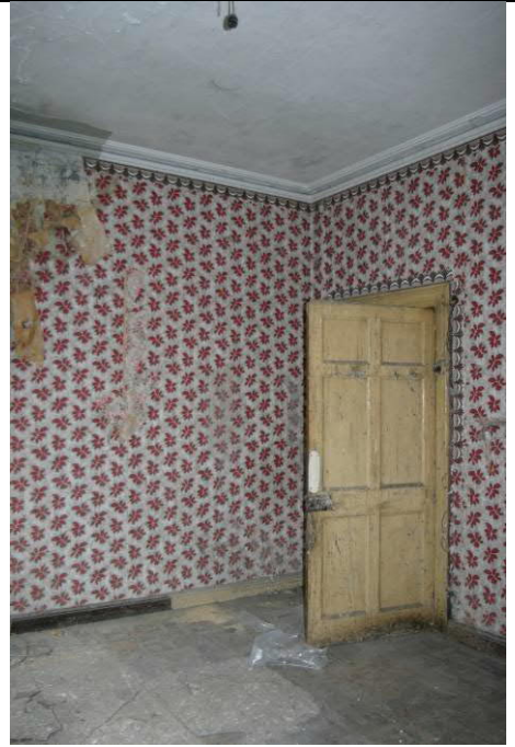
Ceiling & cornice 8 Ellen Street
