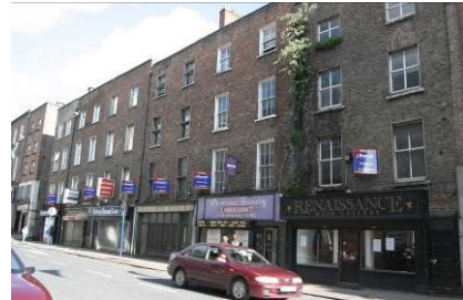
Patricks street Façade
