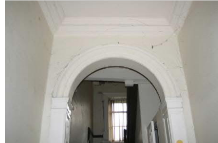
Entrance hall 5 Rutland Street
